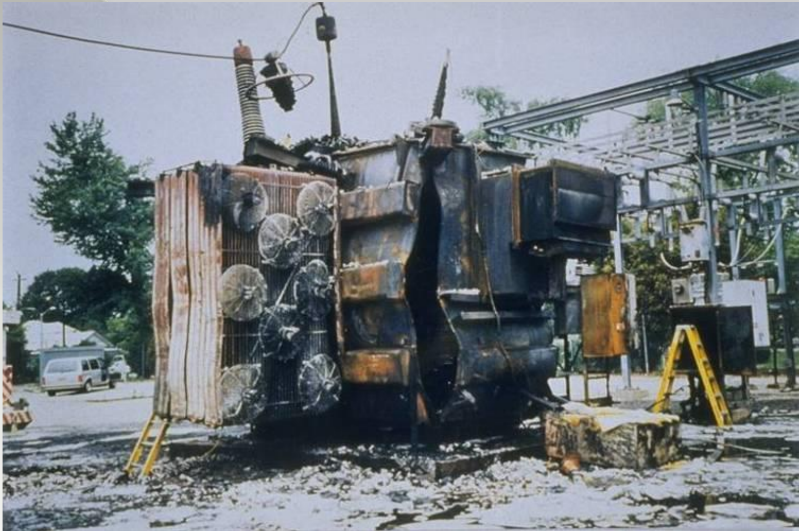
Squirrel Caused Outage – Station Transformer Destroyed
